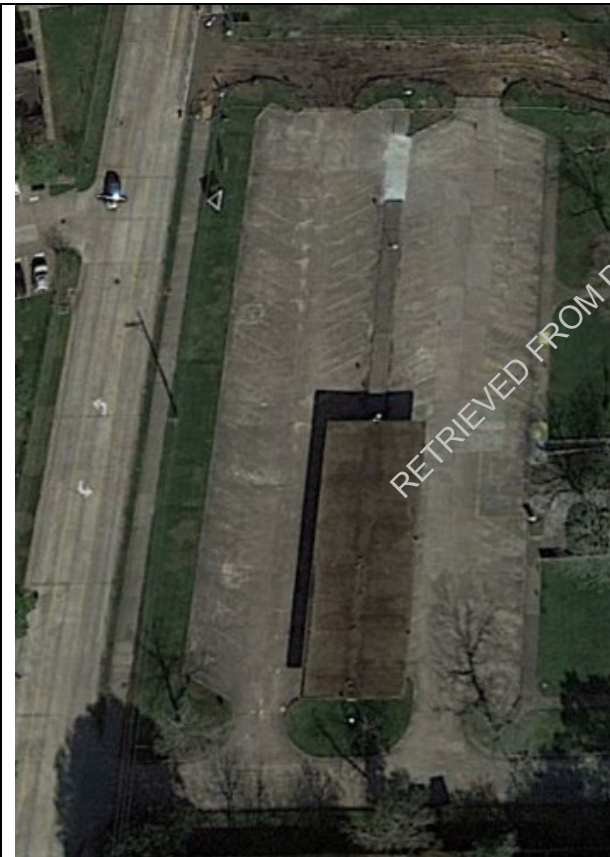
(Above - December 11, 2021 Google Earth image showing north lot construction and open south lot entrance)
